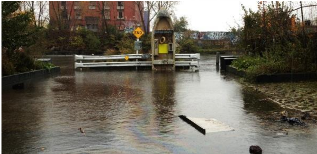
After Hurricane Sandy, 2012
