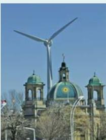
Exhibition Place, on Toronto's waterfront, is host to a 600 kW, 30-storey wind turbine. North America's first urban commercial-scale wind turbine is jointly owned by a local for-profit co-operative (Windshare) and by the City of Toronto's energy utility (Toronto Hydro). The turbine was constructed in 2002, at a total project cost of \$1.8m. It produces around 1000 MWh every year, enough to power approximately 100 homes.
