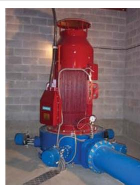
The District of West Vancouver is generating power from its drinking water system, with a 200 kW turbine that replaced a pressure-reducing valve.
